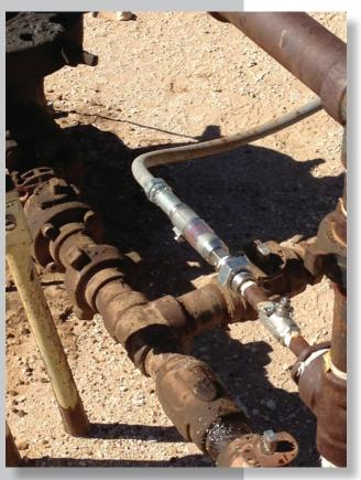
SOR also partnered with a well respected seal manufacturer to create a custom ½" NPT flush diaphragm seal system that allows the 805QS to maintain catalog specifications even with the seal installed. This means the 805QS provides the highest level of protection under varying process conditions.
