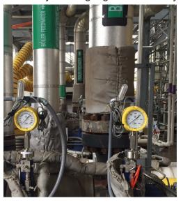
the 815PT and gauge to share the same diaphragm seal process connection. The customer is now fully satisfied with the installed solution as they are now able to read pressure locally with a gauge and offer a 4-20mA output while communicating via HART all in a single efficient and cost effective package.
