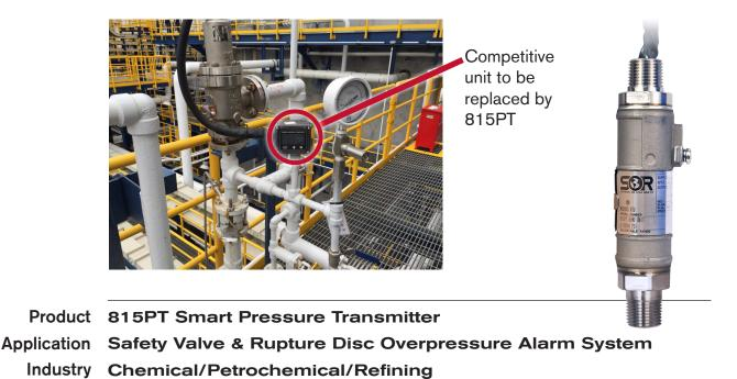
**Challenge** A petrochemical plant was using a competitor's digital pressure switch to monitor overpressure on a safety valve and rupture disc. The unit was giving false alarms which would confuse and waste the customer's time trying to figure out if it was a true alarm.
