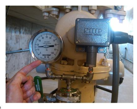
a REOTEMP all welded Diaphragm Seal Assembly and Gauge. The all welded seal assembly allows the customer to isolate the total system, remove it from service, remove the lower housing of the Diaphragm Seal and clean out any clogging without compromising the integrity of the fill. REOTEMP managed the impeccable workmanship with an all welded "Goalpost" T-Assembly. CFMSD hand delivered the first unit and oversaw the installation and testing.
